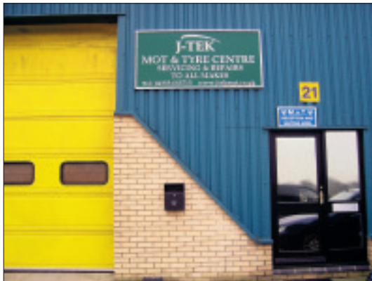
Top facilities: At Lancaster Way Business Park site.
